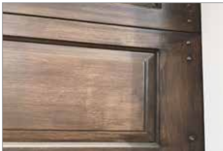
Ends are thru-drilled for carriage bolts
